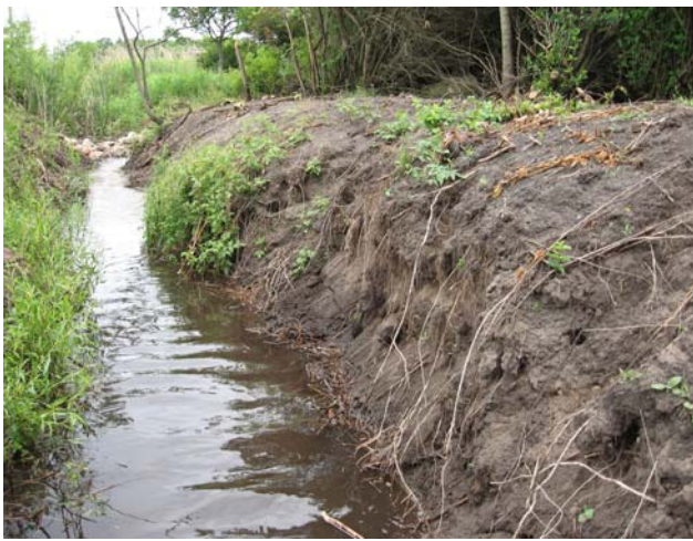
Site BC2 (Before): This eroding streambank was contributing sediment to Bear Creek. The severe slope and sandy conditions were contributing to the bank erosion.
