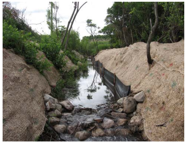
Site BC2 (After): Three (3) check dams were placed along this tributary of Bear Creek; the bank was reshaped, seeded with native grasses and covered with an erosion control blanket.
