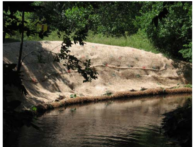
Site 17 (After): Coir (Fiber) Logs were installed to stabilize the toe of the bank. The upper bank was reshaped, seeded with native grasses and covered with an erosion control blanket.
